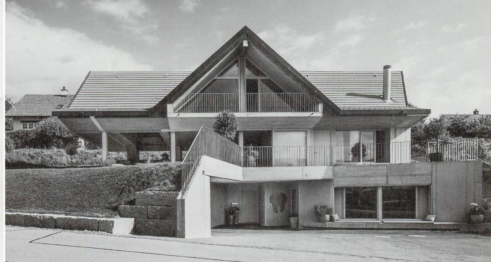
South elevation on street. Dental clinic of owner on basement 街路側、南面。地階はオーナーの歯科クリニック
